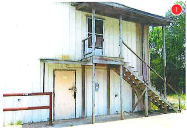
Rear view of large warehouse
