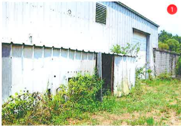
Rear view of large warehouse
