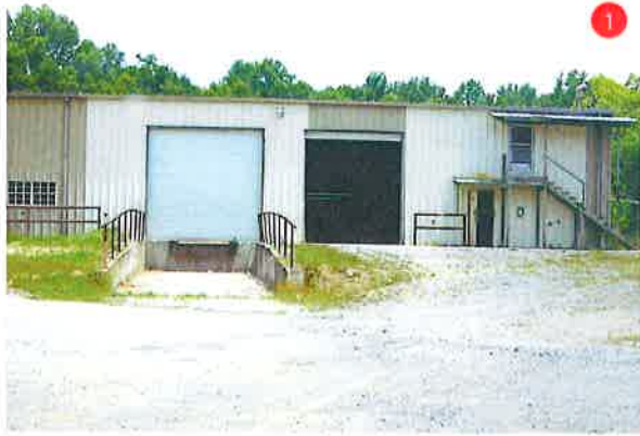
Large warehouse and front loading docks
