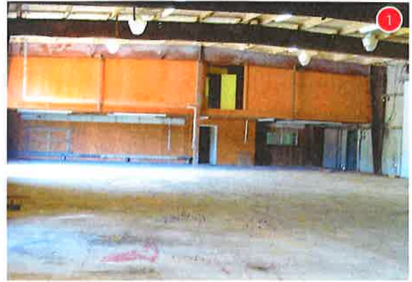
Inside of large warehouse
