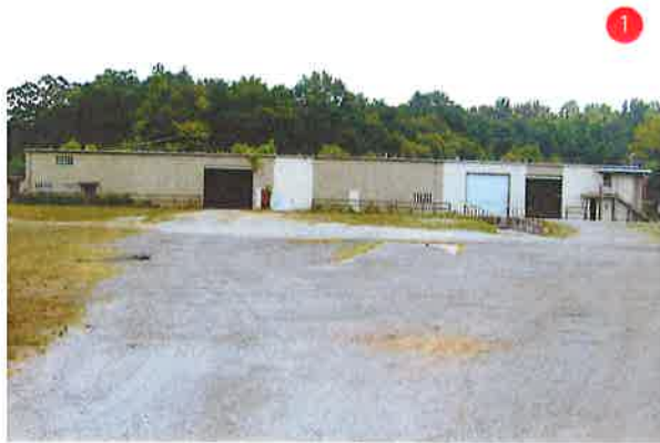
View of large warehouse from road
