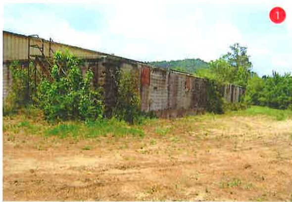
Rear view of large warehouse
